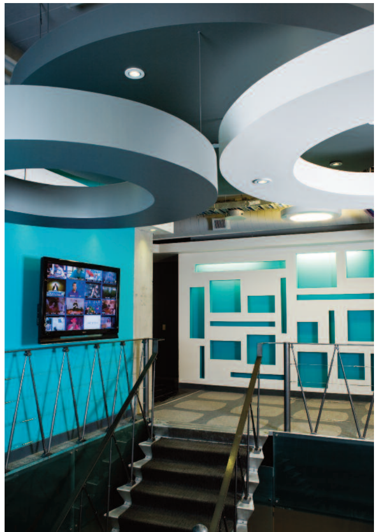
Vivid paint hues and punched drywall partitions inexpensively add some drama and creative ambience to the space for the Design & Graphics department in the 299 Queen Street West building.
